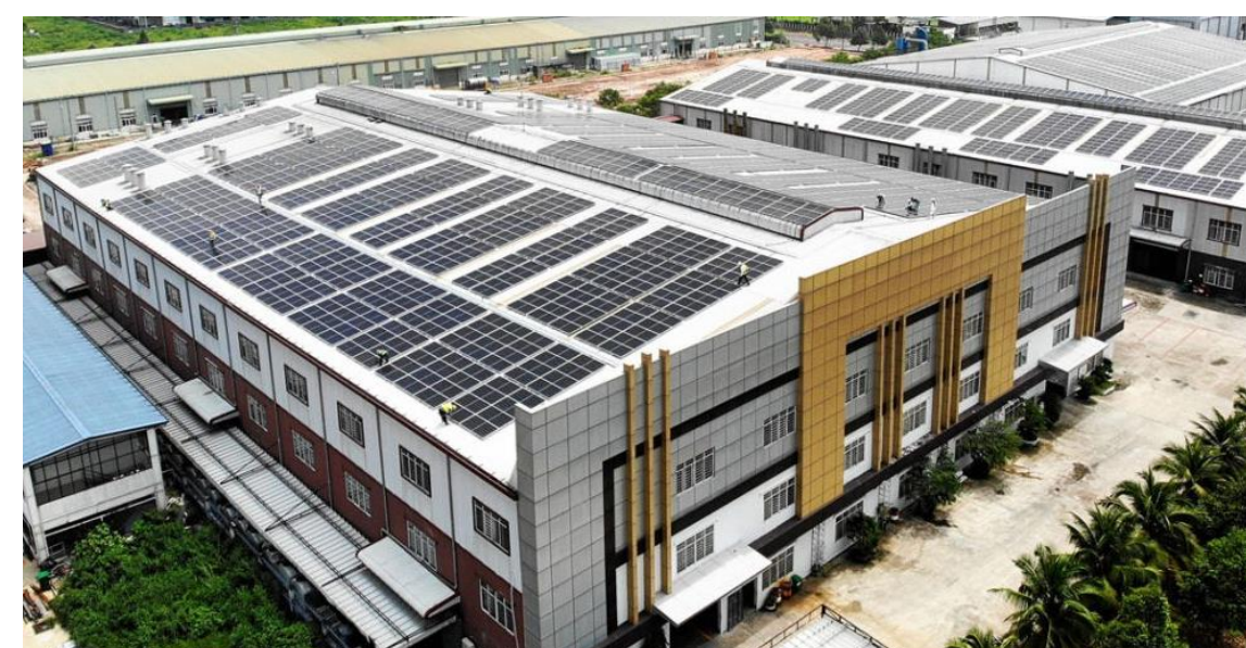
Clean Wood, Binh Duong | 760.32 kWp
