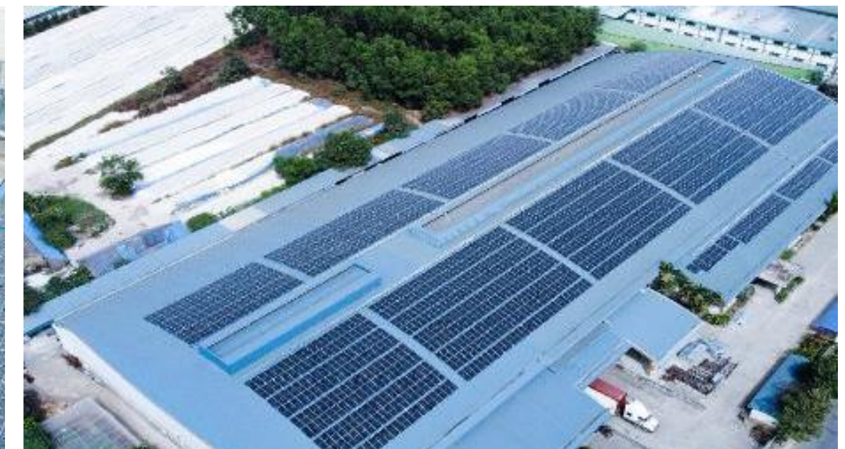
Fabtek, Binh Duong | 1,105.83 kWp
