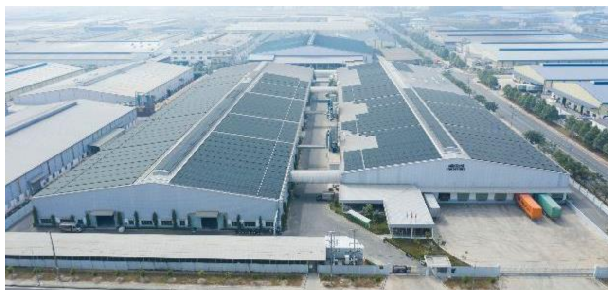
Mekong Furniture, Binh Duong | 3,247.8 kWp
