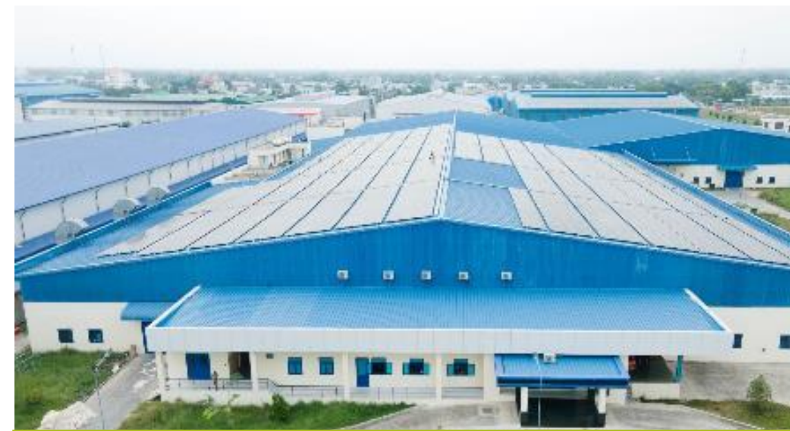
Viet Phu, Long An | 999.68 kWp
