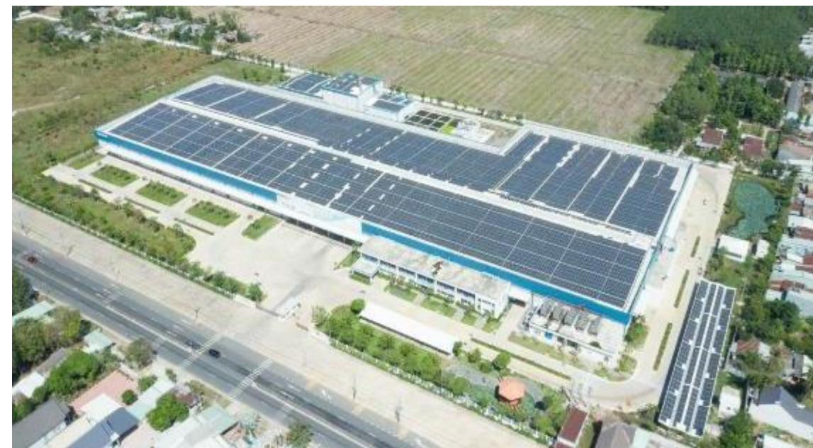
Tanifood, Tay Ninh | 5,125 kWp
