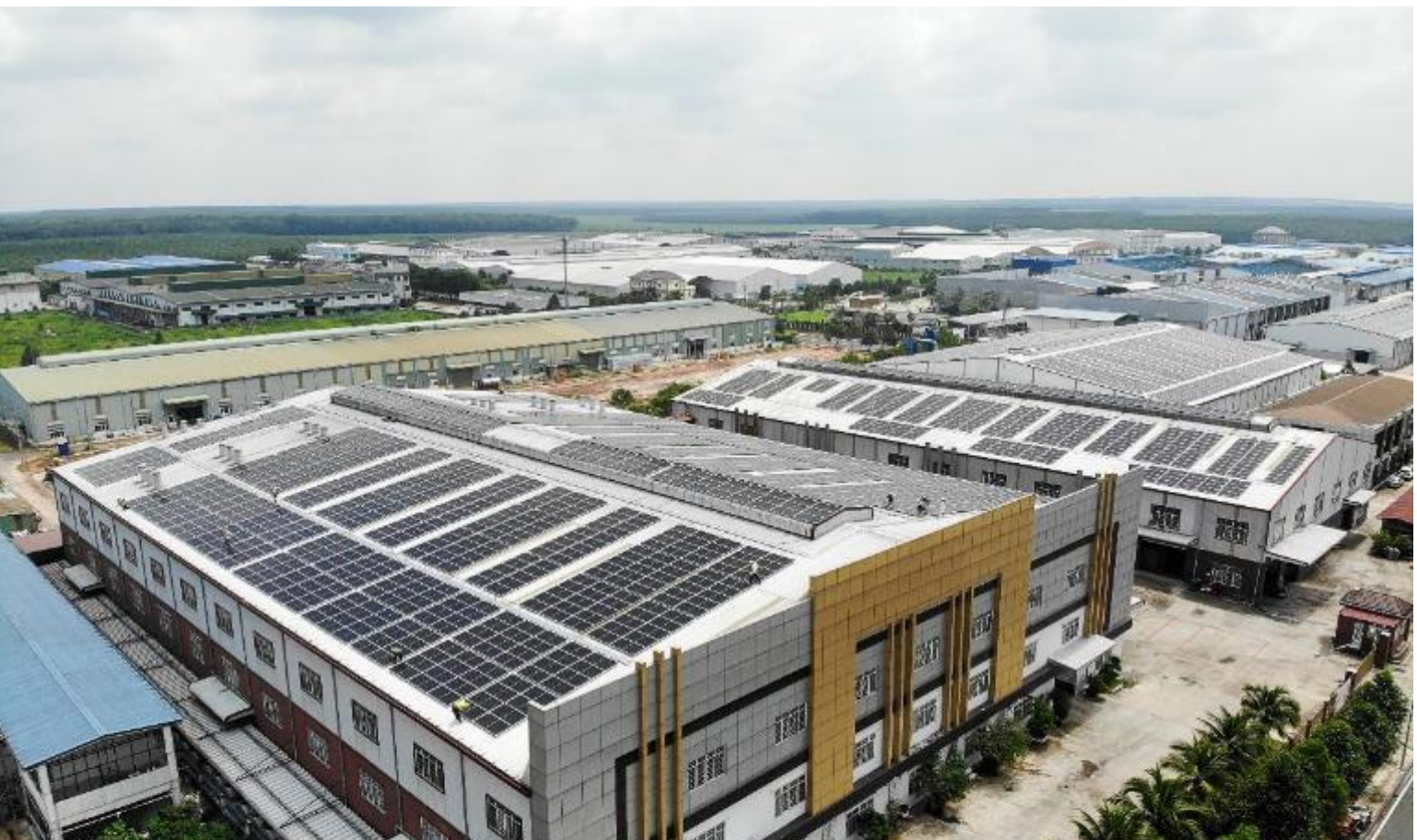
Clean Wood | 760.32 kWp
