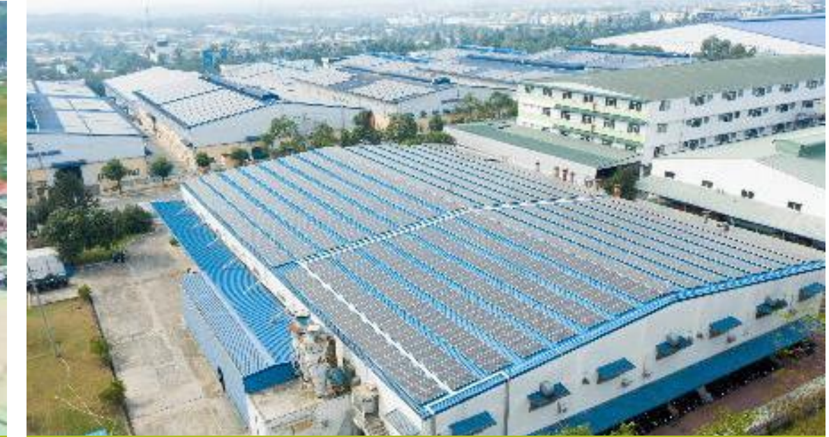
Daigaku, Binh Duong | 421.98 kWp
