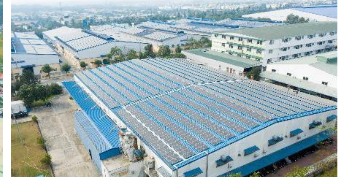
Daigaku, Binh Duong | 421.98 kWp
