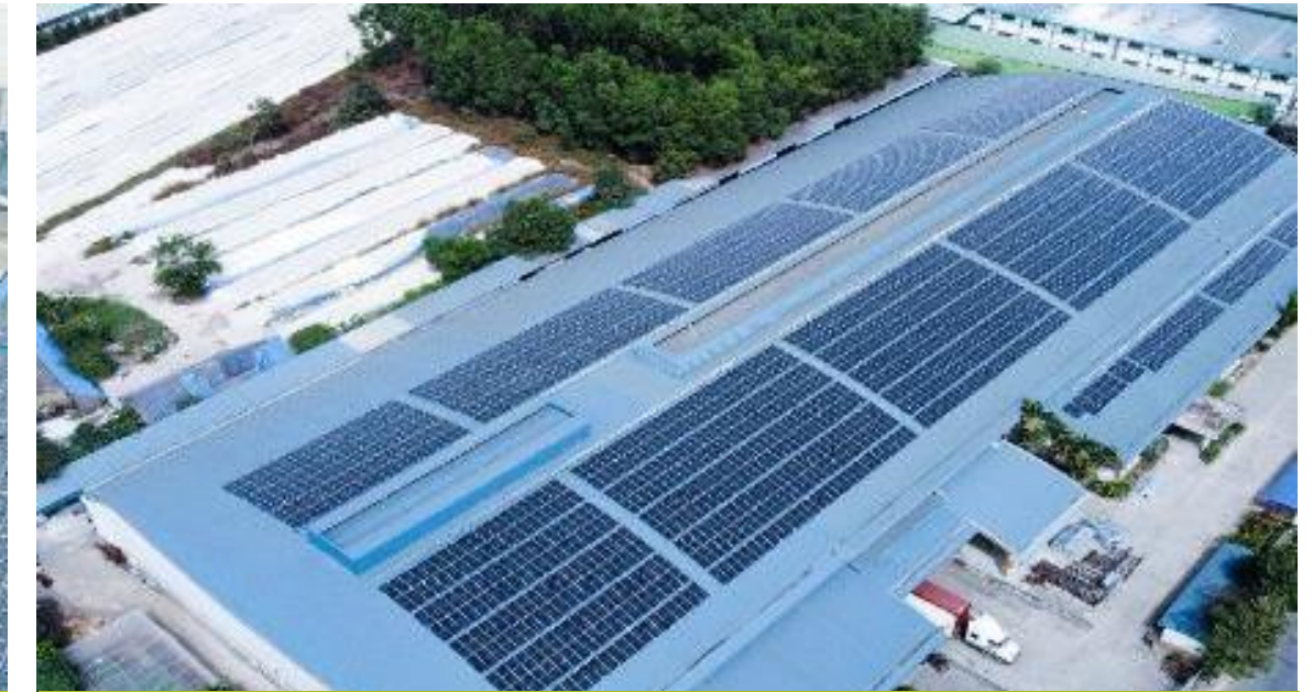
Fabtek, Binh Duong | 1,105.83 kWp
