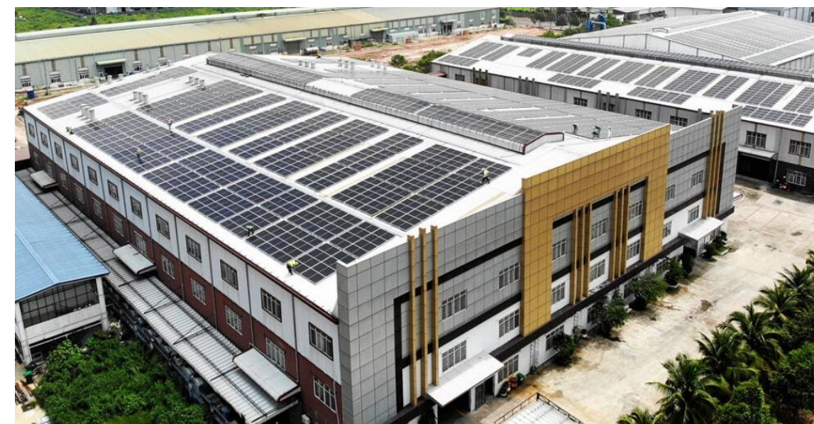
Clean Wood, Binh Duong | 760.32 kWp
