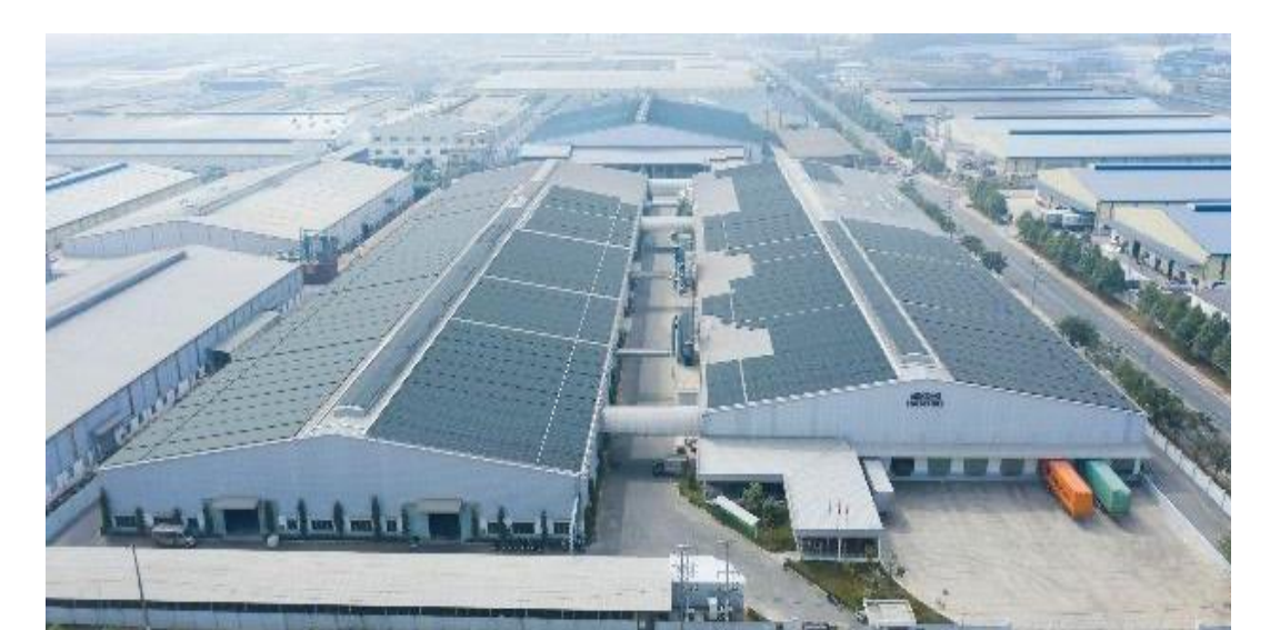
Mekong Furniture | 3,247 kWp
