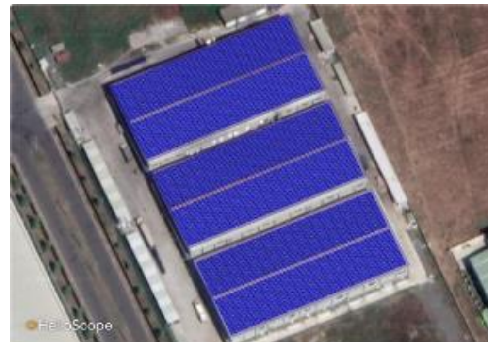
DKFS, Long An | 1,630 kWp
