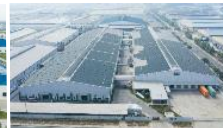
Mekong Furniture | 3,247.8 kWp
